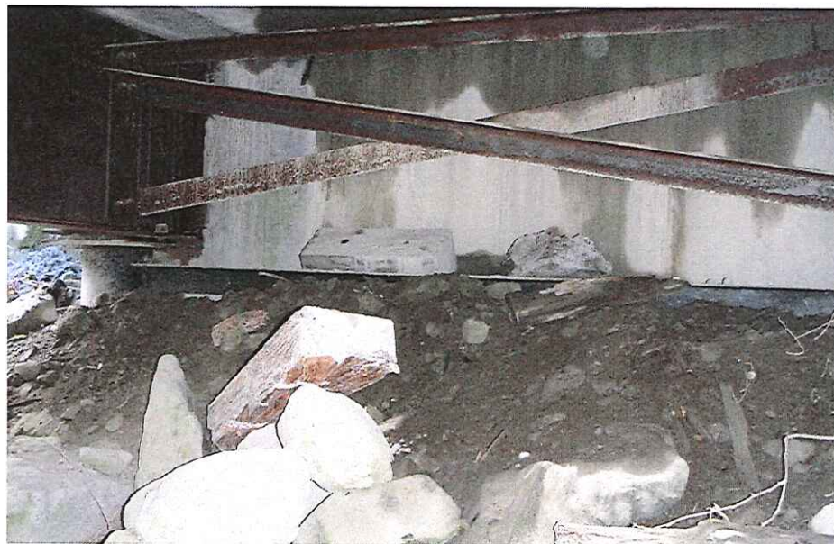
CK-2092 Abutment Right Bank #2
