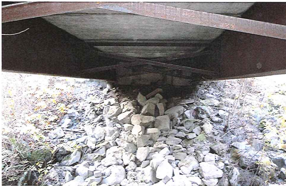
CK-2092 Abutment Right Bank
