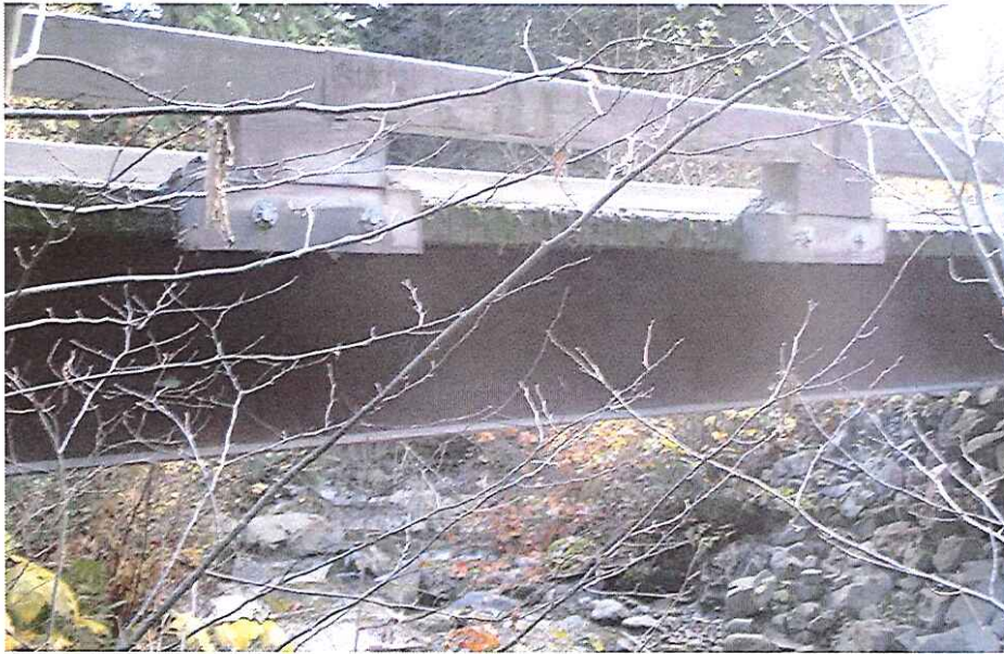
CK-2092 Crossing Upstream
