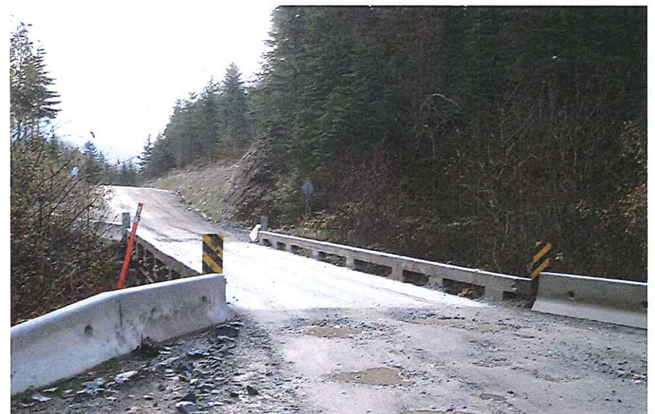
CK-2092 Approach Left Bank
