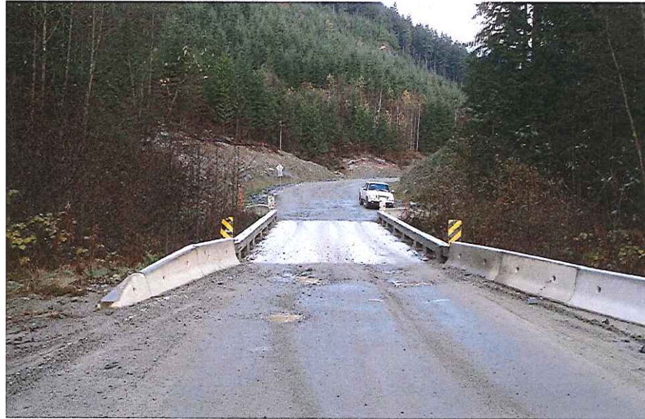
CK-2092 Approach Right Bank
